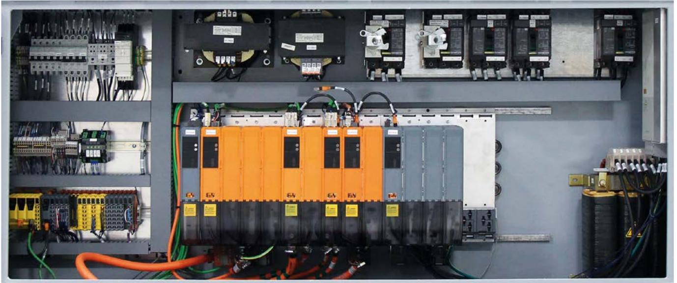
Pairing B&R's Power Panel technology with ACOPoS multi drives reduces the number of necessary components and saves cabinet space, resulting in a very clean and simple cabinet layout.
