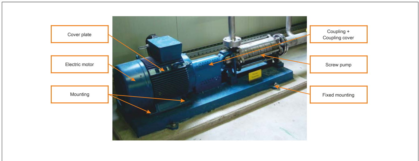
Figure 82: Structure of a pump drive
