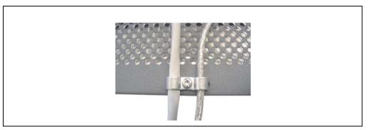
Figure 50: Mounting the cable clamps
