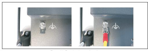
Figure 75: Functional grounding clip
